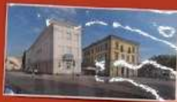
Building nr 28 and 29 on Tartu Kesklinn plats. Nr 28 is an old the Leaning House of Tartu, built in 1716. One side of the house is foundation supported by the old brick wall and the other side by concrete piles. This is the reason why the house is leaning eastward. Nr 29 is iron building, built in 1870-1874.
